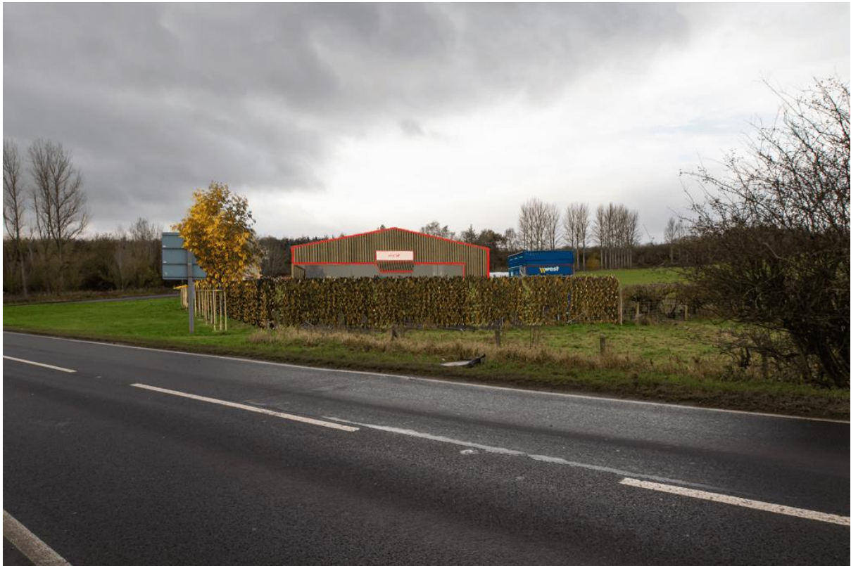
View from A68 looking south west
