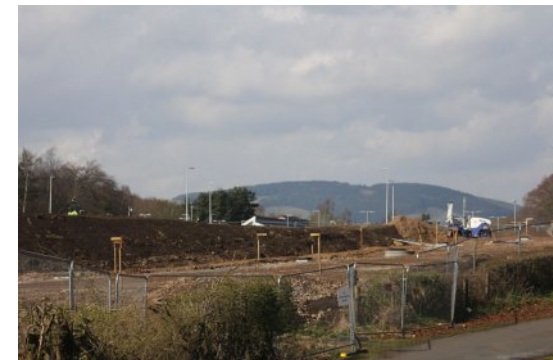
Ongoing infrastructure development
